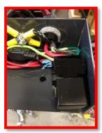
3. Inline fuse. Found inside electrical box. (7.5amp automotive type 2 prong fuse) <u>https://www.youtube.com/watch?v=JZZmYQtybAE</u> replacing fuse
